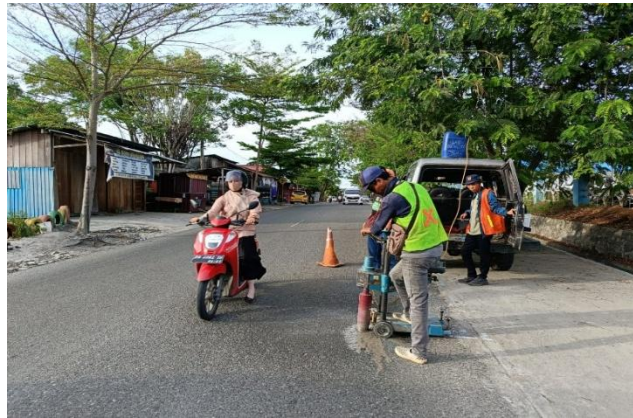
Gambar 3. 4 Proses pengambilan sampel core drill
